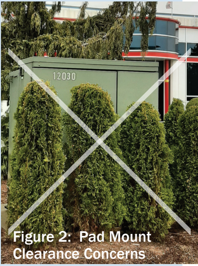
Figure 1: Clearances to Pad Mounted Equipment
